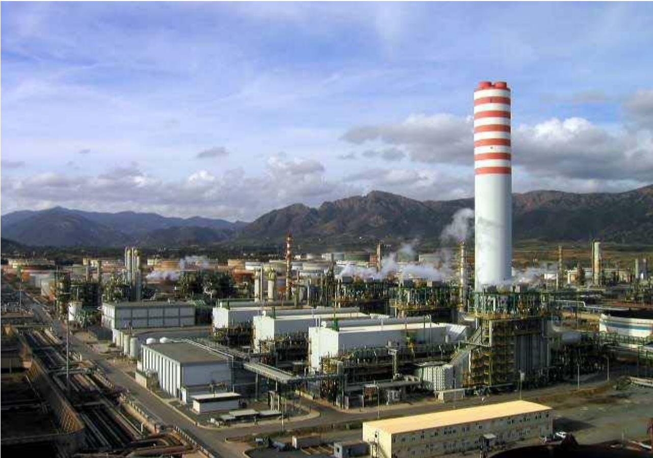
IGCC power plant overview
